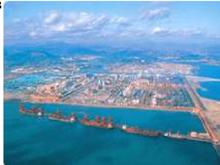
Kwangyang Steel Plant
